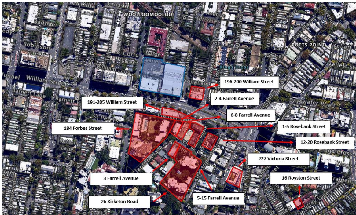
Figure 51: Aerial photograph of the subject site and surrounding properties raising view loss concern
