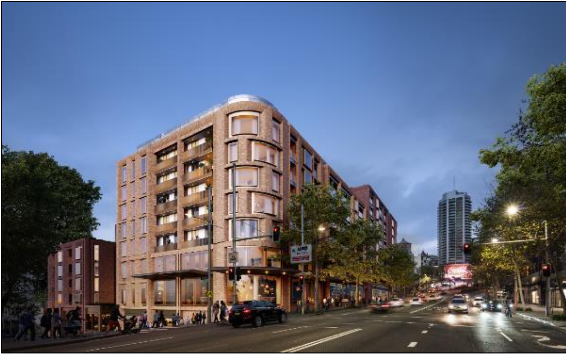
Figure 22: Indicative proposed photomontage, viewed from the corner of Willam and Forbes Streets
