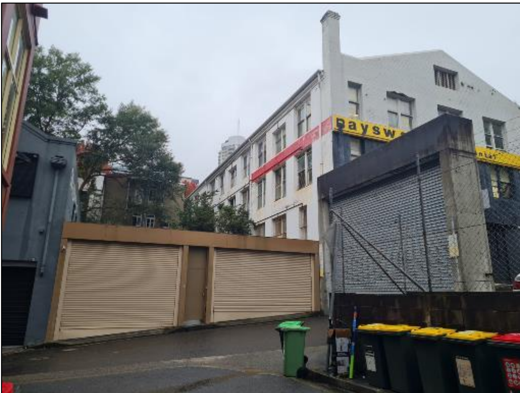
Figure 10: The site viewed from the end of Judge Lane, looking east
