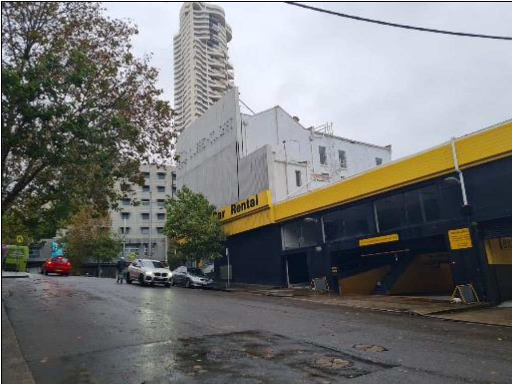
Figure 11: The site viewed from Dowling Street, looking south-west
