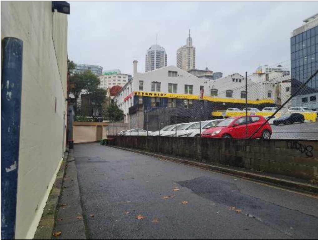
Figure 9: The site viewed from Judge Lane, looking east
