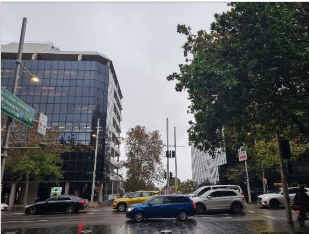
Figure 15: Commercial building at 150-162 William Street looking north
